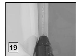
19. After achieving alignment; from the inside, drill four 3.0 mm holes, starting 30mm from the ends and then equally spaced down the screw indicator line on the Return starter. The screw indicator line is a **“Vee” groove that runs down the length on the inside faces of the Return Starter, Door Starter and 90° corner post to ensure correct position of screws in relation to other components.**
