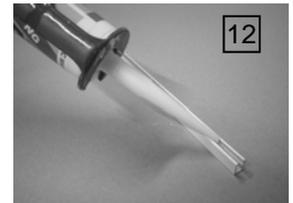
12. Apply a small continuous bead of NG Silicone sealant into the bottom of the Return sill channel. **Do not fill** the channel with silicone as this will be excessive and the majority will ooze out making cleanup difficult
