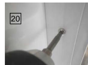
20. Secure with the No.6x10mm stainless steel screws supplied.
